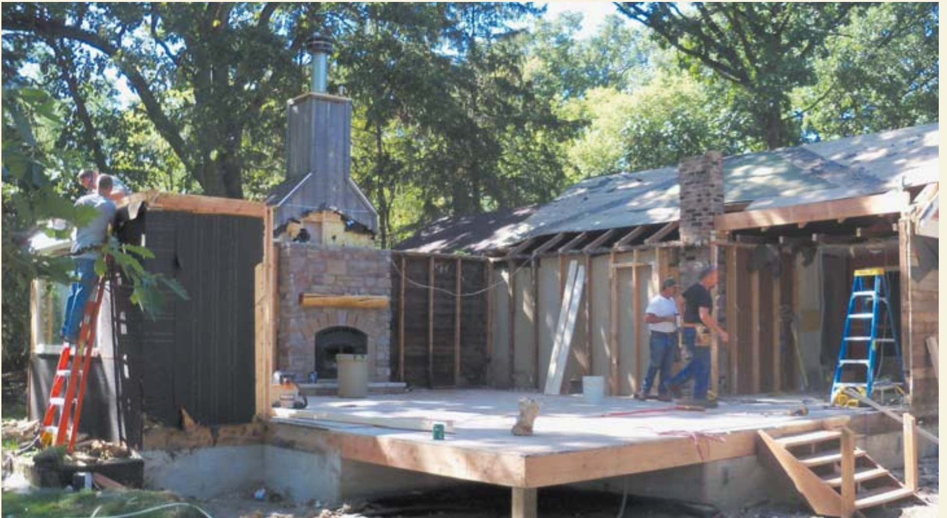
In just a weekend, leaving the fireplace having an idea, the Utsches tore off the old roof and built new walls and a new roof.
